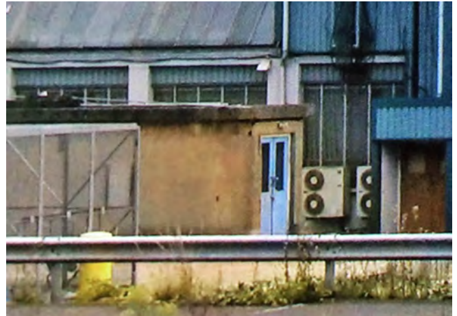
The surface blockhouse was the entrance to the tunnels.
